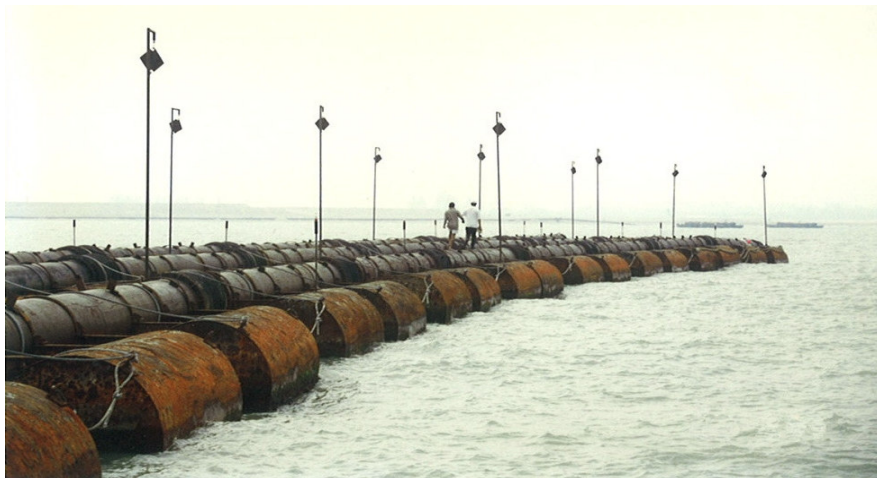
Floating Pipelines used as Artificial Barrier to minimise destructive sea waves that erodes the coast
