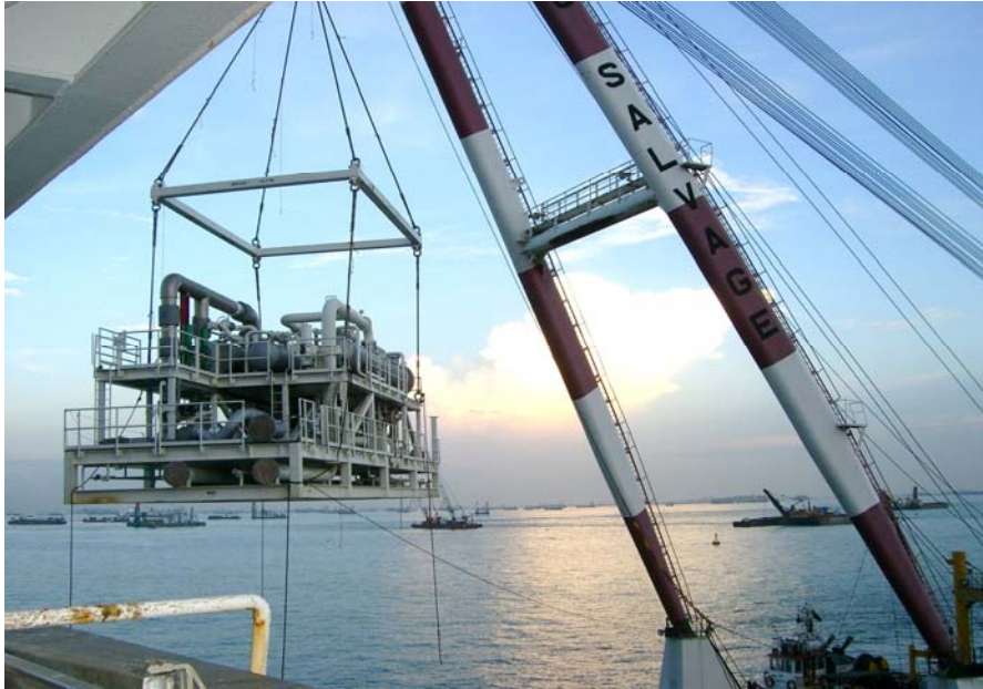
Transportation of Module Dehydrators loaded onto Barge Winstar II (180ft x 50ft x 10ft)
